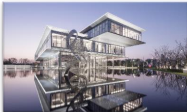
Hangzhou Central Mansion
