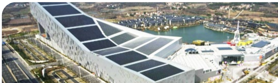
Photovoltaic System Installation at Wuhan Bonski
